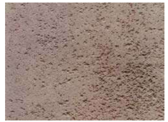
Condition D Blasted to Sa2.5
