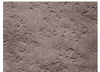
Condition D Blasted to Sa3
